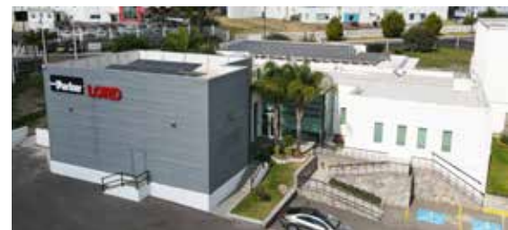
Parker's Querétaro, Mexico facility is saving approximately 60 MT CO 2 annually by using power from rooftop solar panels, and several locations worldwide are currently pursuing their own solar installations.
